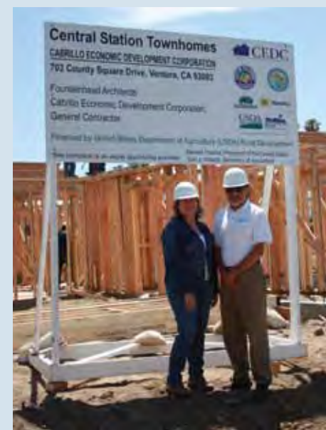
Fillmore Mayor Patti Walker took a few minutes to visit the site of Central Station, a 29-home development which began construction in October last year. It will feature eight for-sale townhomes and 21 apartment homes for farm workers.
